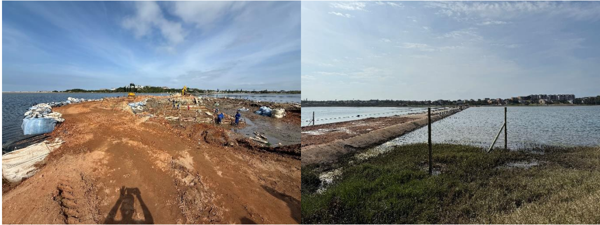
Figure 4.1: Maintenance and repairs currently underway on the causeway crossing the Seekoei estuary
