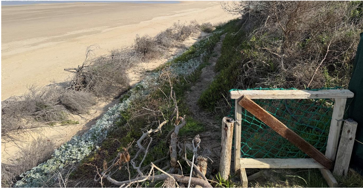
Figure 4.7: An example of where an informal footpath is exacerbating dune erosion
