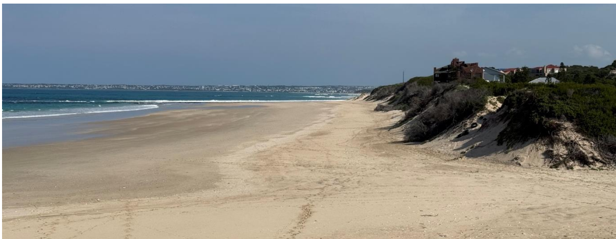
Figure 4.18: An example of coastal erosion where the foredune is being eroded by storm surges
