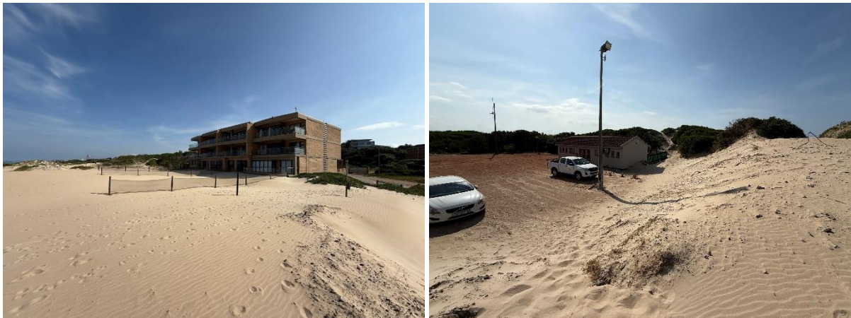
Figure 4.17: Examples where sand inundation is affecting properties and infrastructure located within the LAZ.
